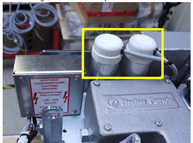
Fig. 3.2.5-16: Booster capacitors 120V/60Hz
