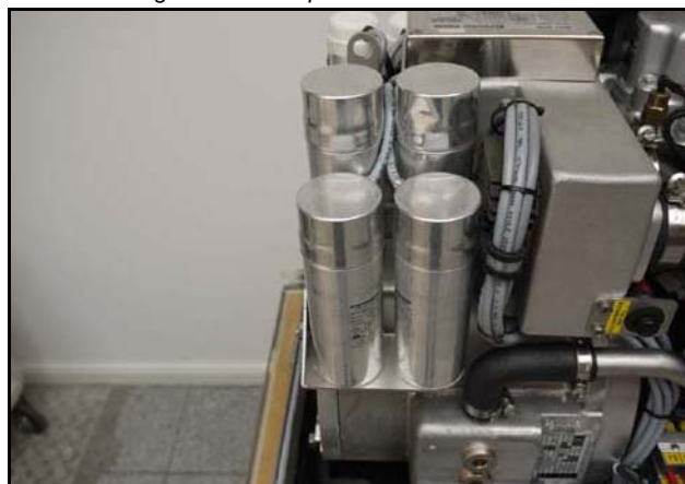
Fig. 7.12.4-2: Capacitors for the excitation
