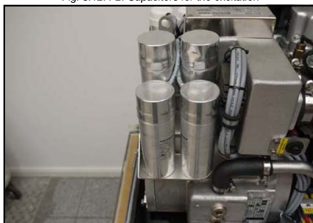
Fig. 5.12.4-2: Capacitors for the excitation
