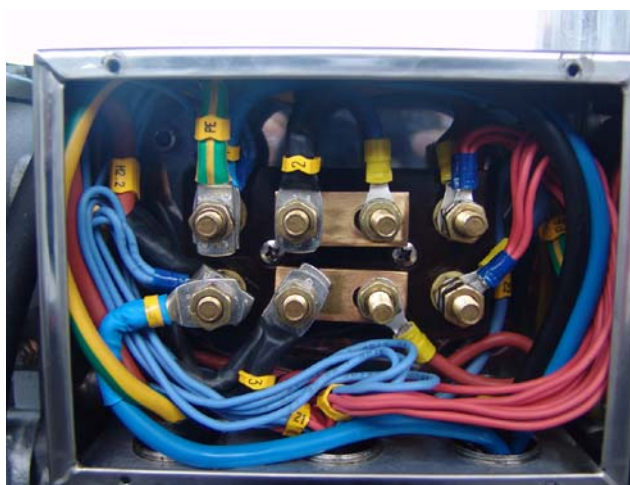
Fig. A.42: Generator power terminal box 120V/60Hz
